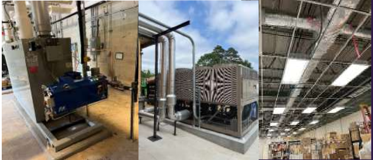
Boiler, Chiller and Fan Coils Commissioned at Ravenel Center on 9th May 2025
